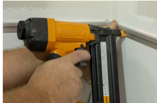
16-18 gauge 1" nails used to hold trim
