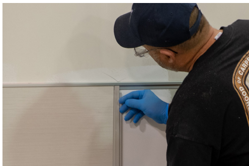
Install next trim
