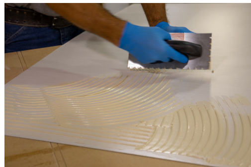
Apply adhesive. 100% adhesive coverage required.
