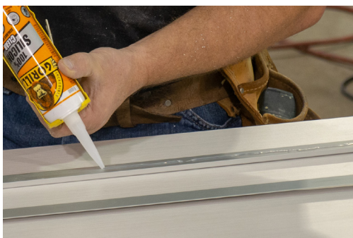
Use 100% clear silicone to adhere trim
